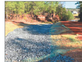
A section of dirt road restored with best management practices 1
