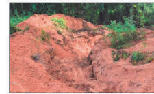
A pile of sediment eroding from a dirt road 1
