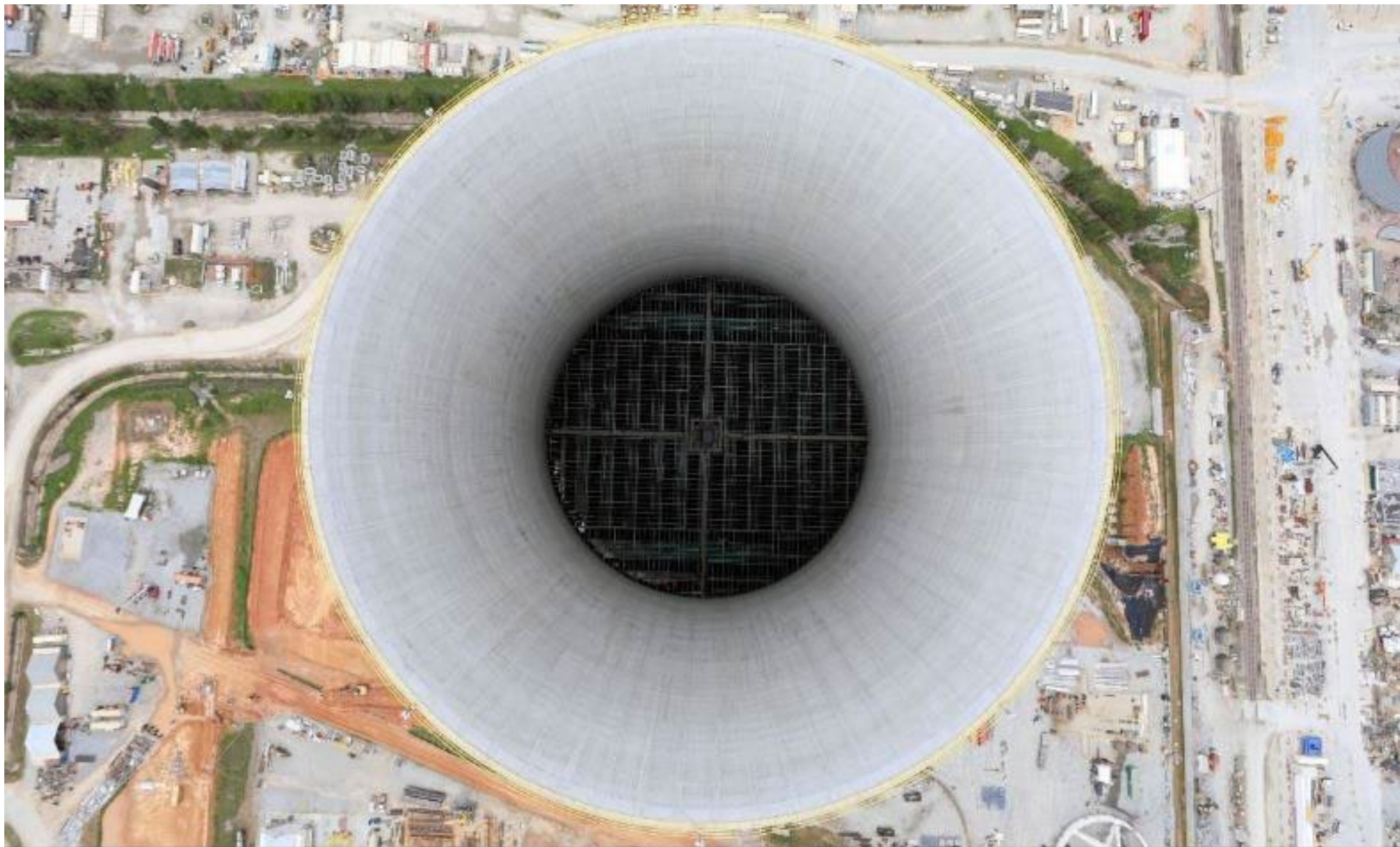
An aerial view looking inside the Vogtle Unit 4 cooling tower.
