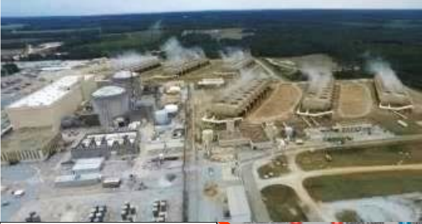
Plant Farley 2 PWR Units (1977, '81) 950 mw each 1,900 mw total
