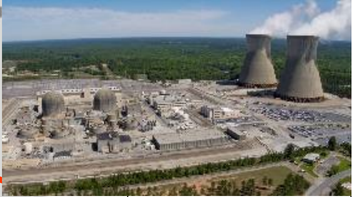
Plant Vogtle 2 PWR Units (1987, '89) 1240 mw each 2480 mw total
