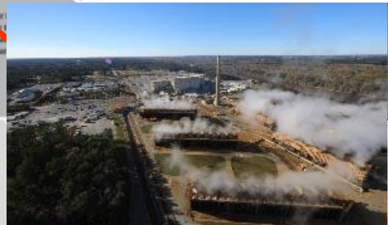
Plant Hatch 2 BWR units 1975 & '79 924 mw each 1848 mw total
