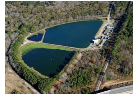
City of Pooler WWTP Membrane Bioreactor Upgrades
