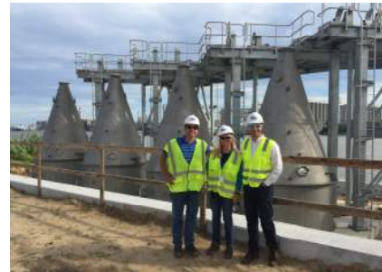
Savannah River Dissolved Oxygen Facility
